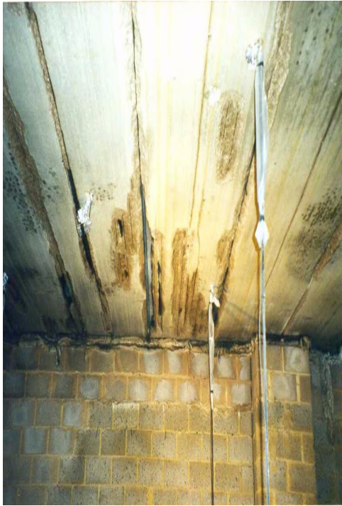
Figure 1 Spalling
