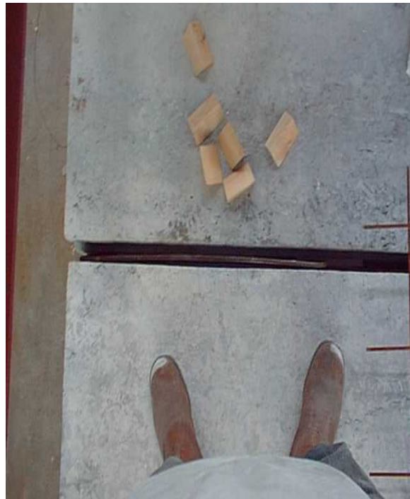
Figure 6 hooked bar over edge beam
