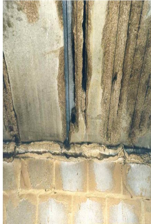
Figure 2 exposed reinforcement
