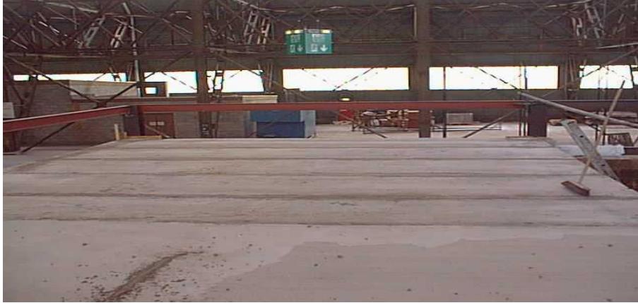
Figure 7 joints filled – slab B
