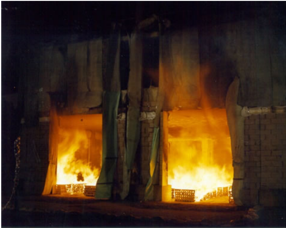
Figure 6 Fire test (Note the start of the spalling of the concrete soffit)
