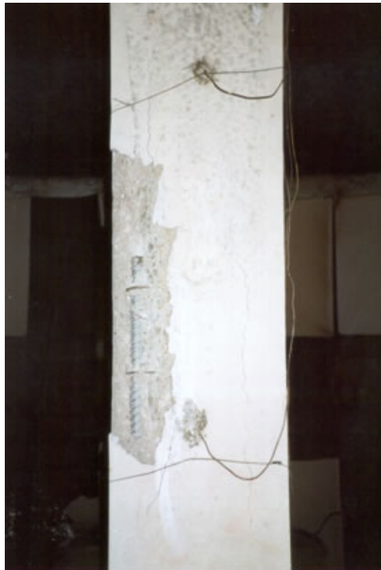
Figure 22 Removal of outer (corner) concrete on column C3
